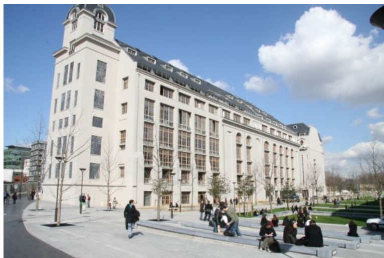
Figure 1: Location of the refurbished 20 th century industrial building where University Paris7 – Denis Diderot is newly installed and where meeting took place.
